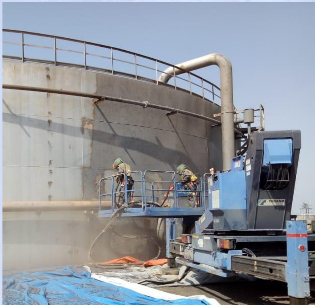
Sand Blasting & Painting Tank - Basra Iraq (Exxon Mobil)
