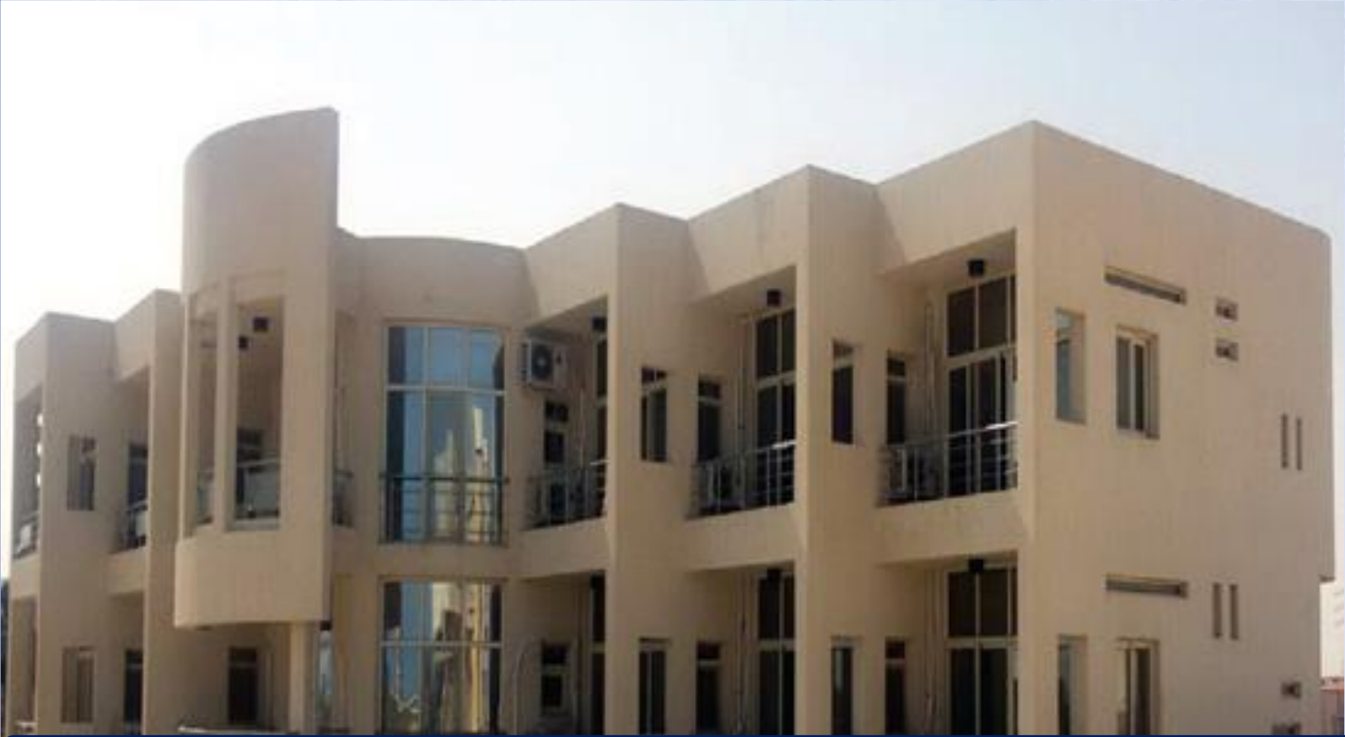
Construction of VIP Building -WEPCO
