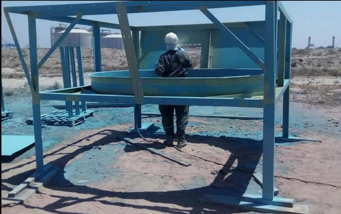
Fabrications, Sandblasting & Painting for Cooler Turbine UGDC
