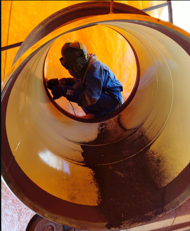
Grinding Works for Isolation Joint 36"- WEPCO (ElHamra site)
