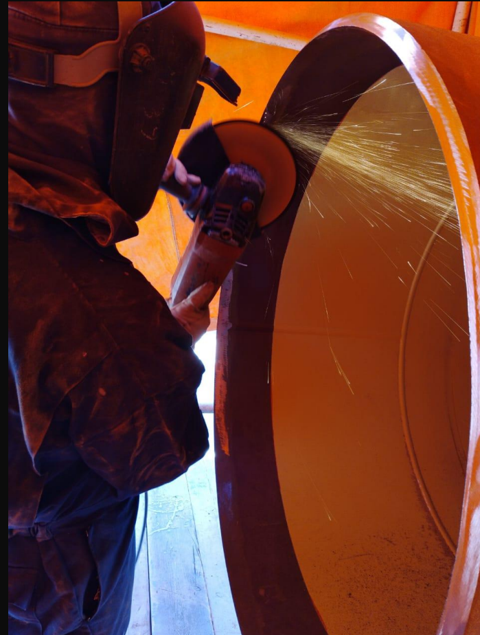
Grinding Works for Isolation Joint 36"- WEPCO (ElHamra site)
