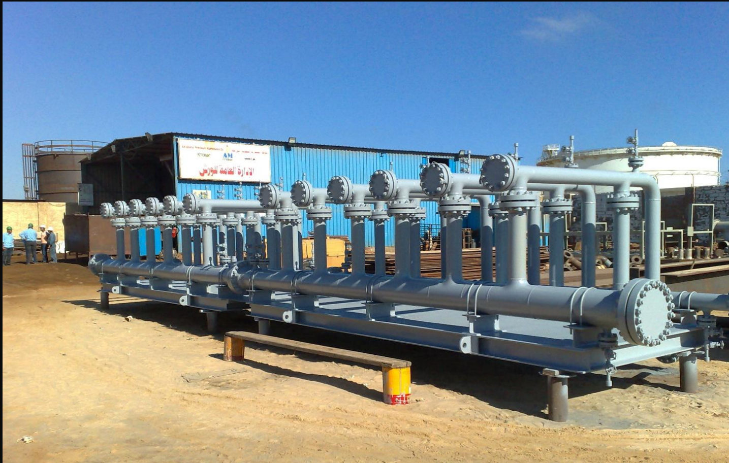
Fabrication & Installation of Manifolds – Workshop Yard
