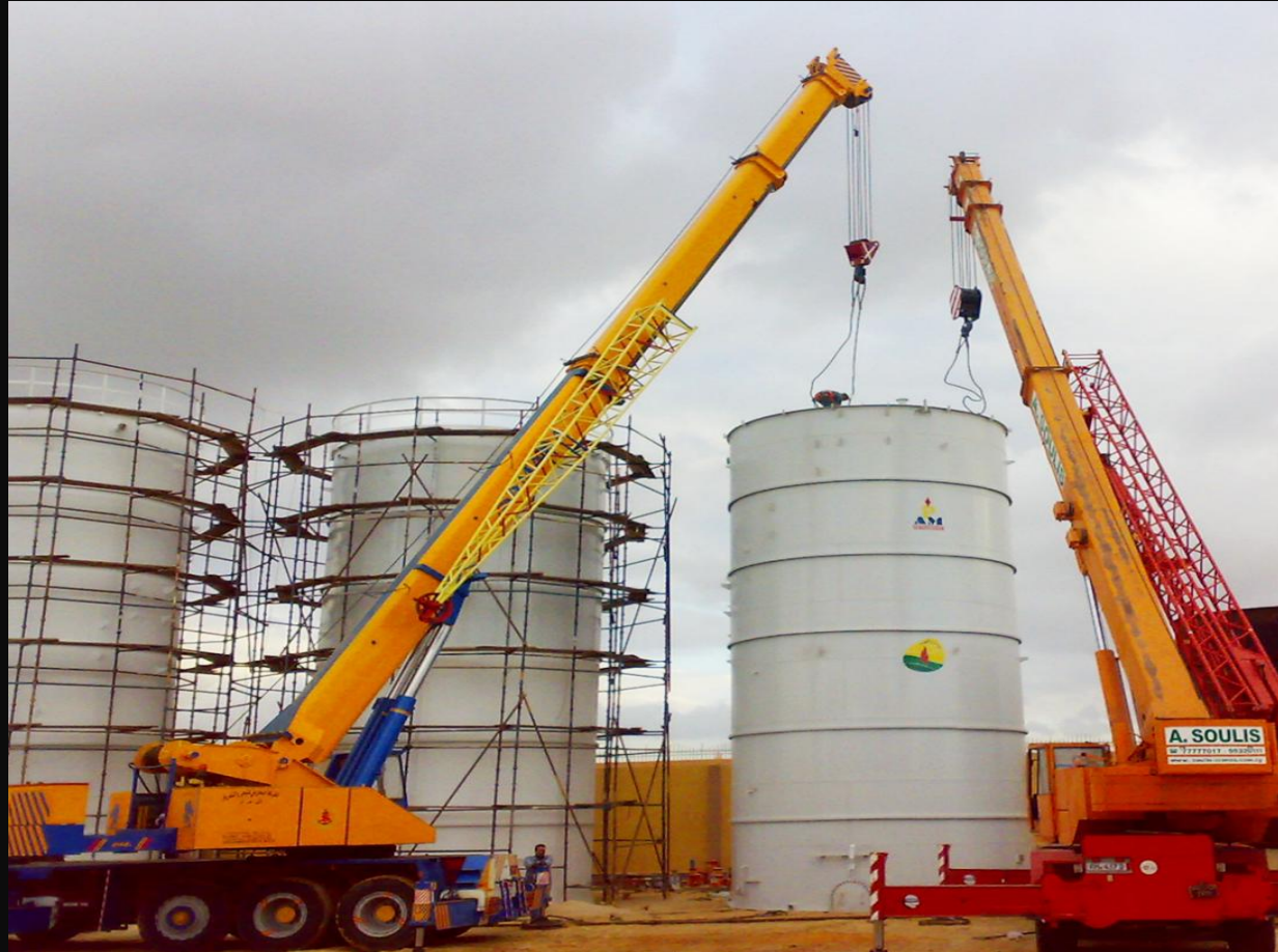
Tanks Fabrication - Petroshahd
