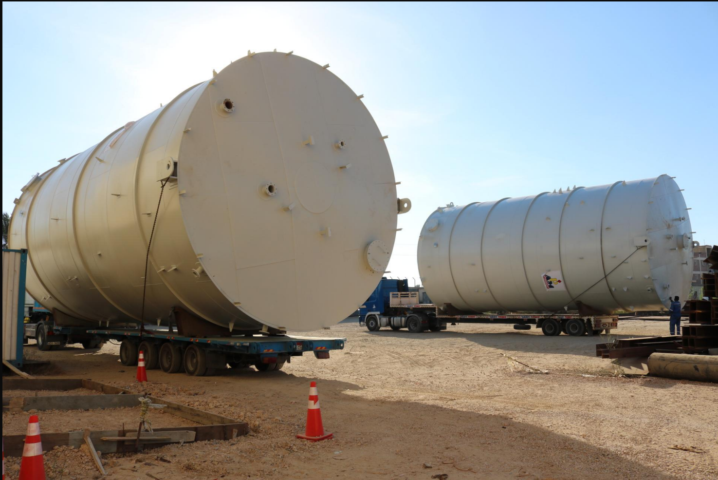
Tanks Fabrication - Qarun
