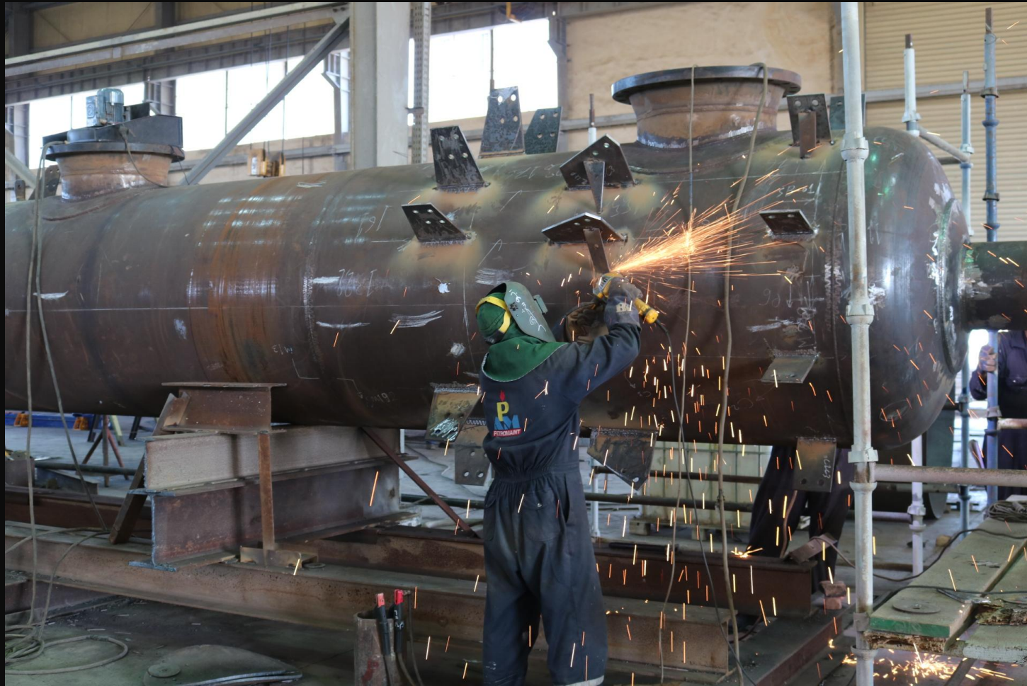
Process equipment & process vessels - Workshop Yard
