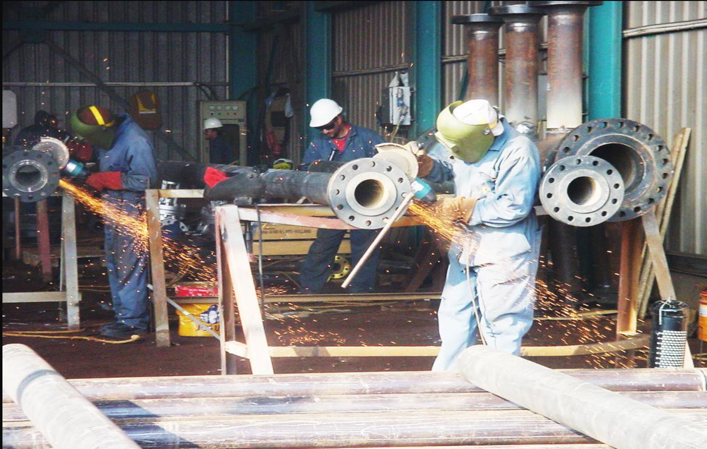
Piping Fabrications – workshop yard
