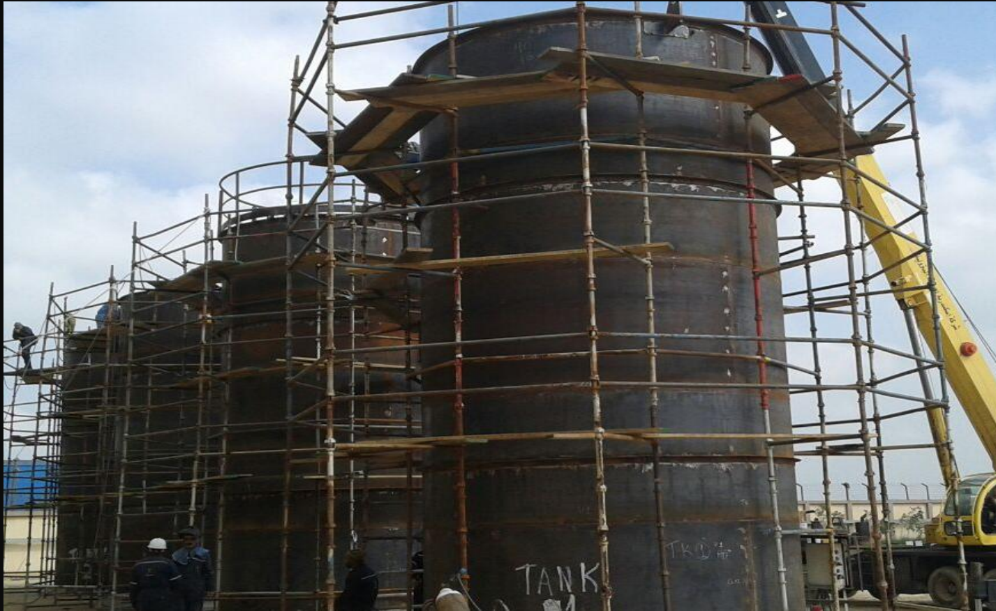
Tanks Fabrications – Qarun
