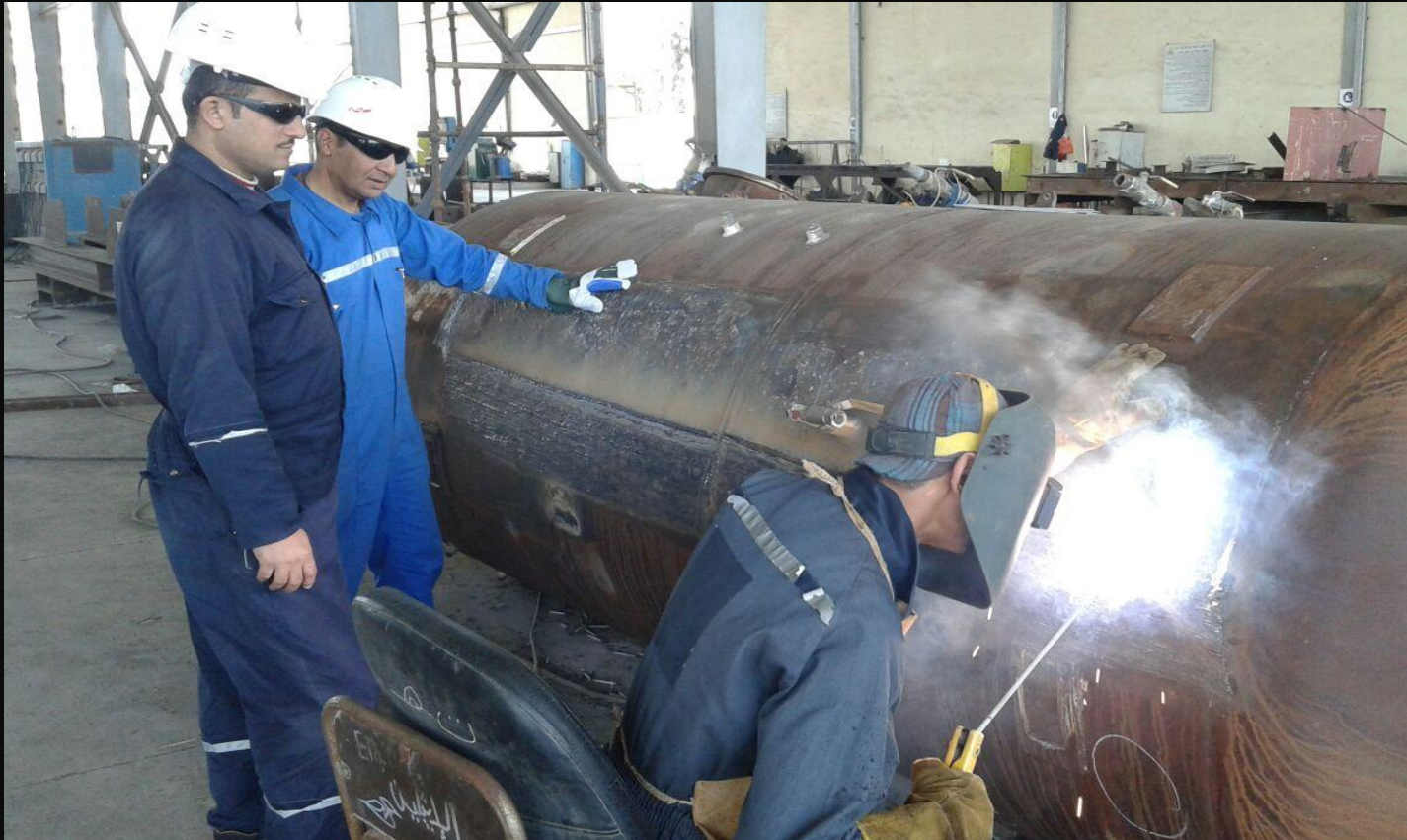
Vessel welding - Workshop Yard
