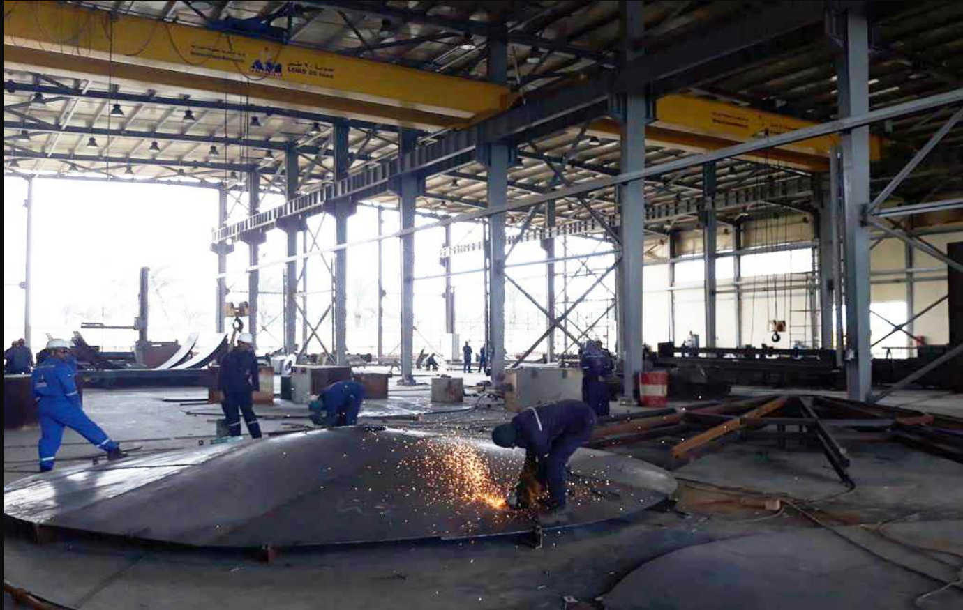
Tank Roof fabrication – Workshop Yard
